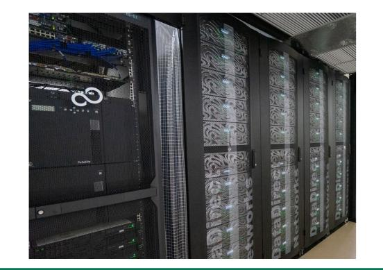
Consists of 30 PB HDD RAID storage (Hot storage) and optical disk archive system for long-term data archival (Cold storage).
